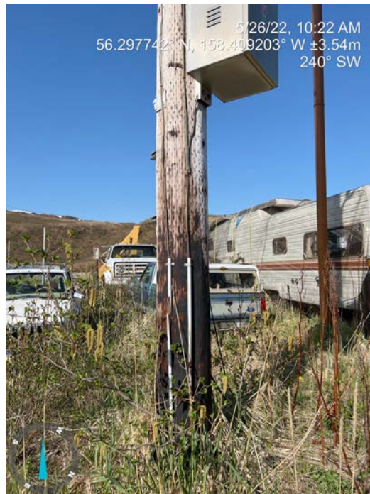
Pole Foundation 1 of 2
