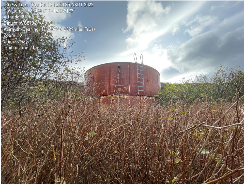
Old East Side Water Storage Tank
