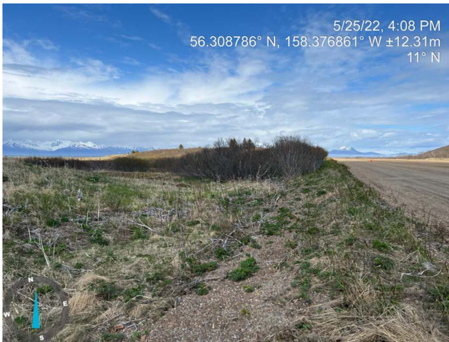
Shoreside Runway Embankment 2 of 2
