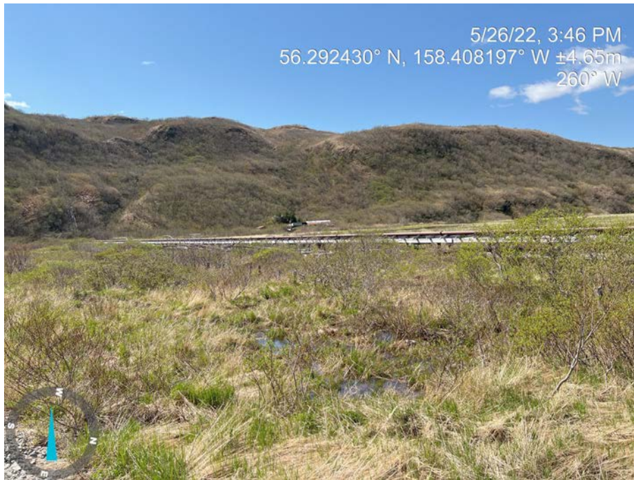
Water Trestle 1 of 1
