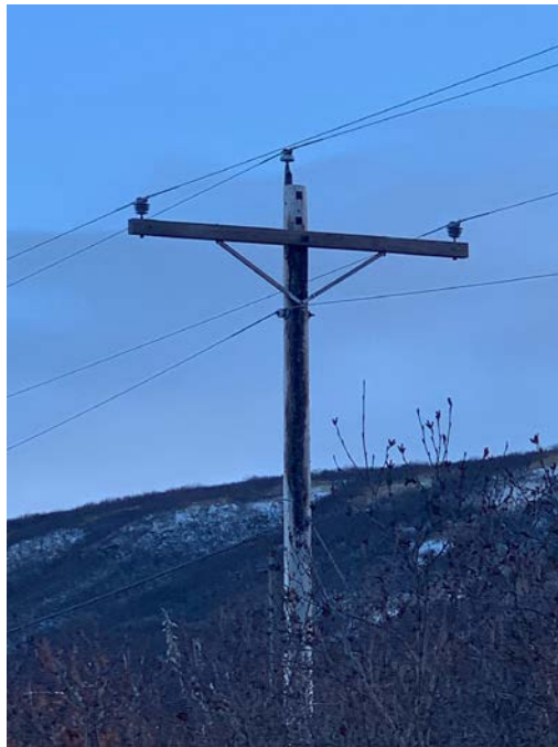
14 - New Cross Member from Prior Fire
