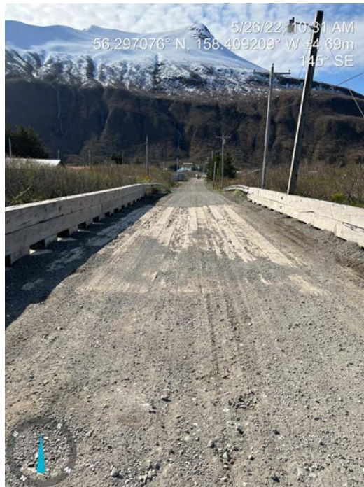
Chignik Creek Bridge 1 of 2
