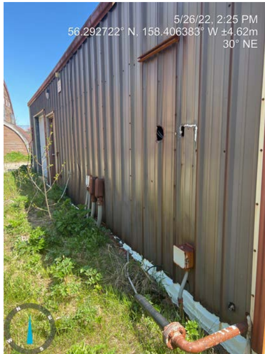
Damaged Siding
