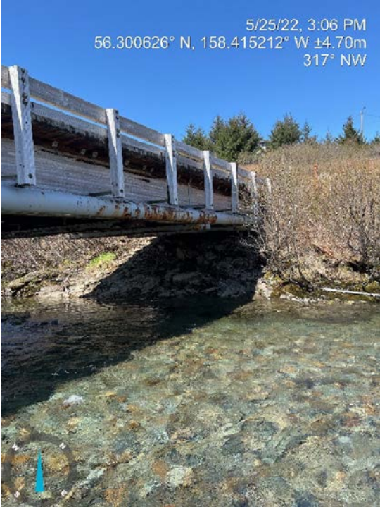
North Side Abutment
