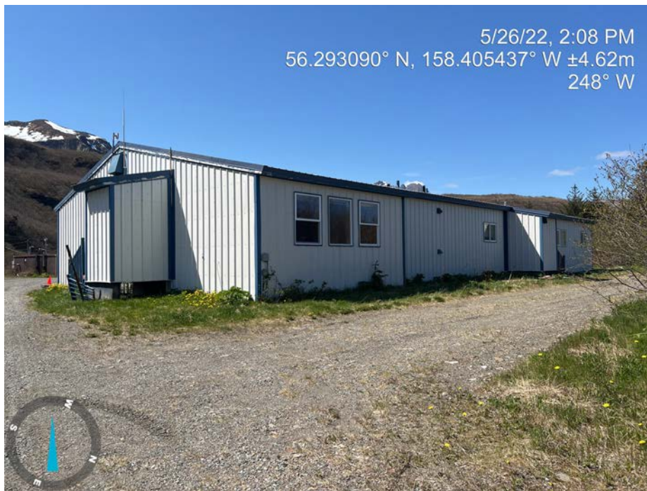
North Elevation 1 of 2
