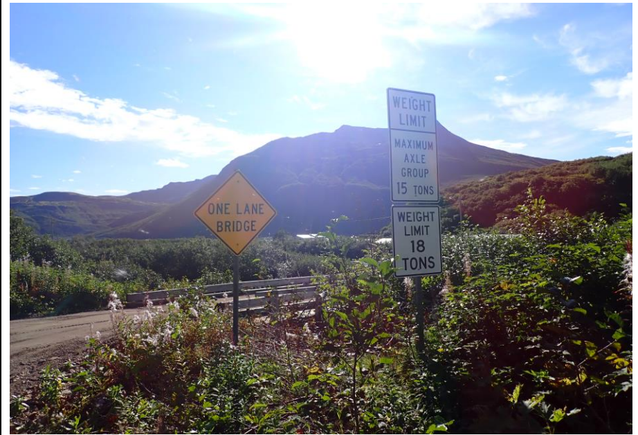
Bridge No. 1764 Br. Name Indian Creek Date 09/21/22 Inspector David McAdoo / Javier De Leon Frame 30 FE US Signage File P9210419.jpg
