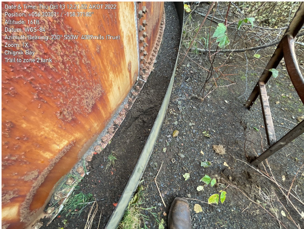
Old East Side Water Storage Tank Foundation
