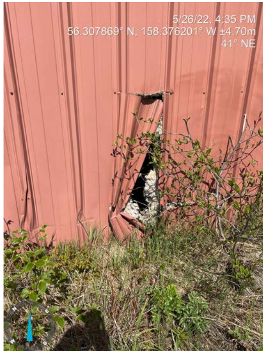
Damaged Siding
