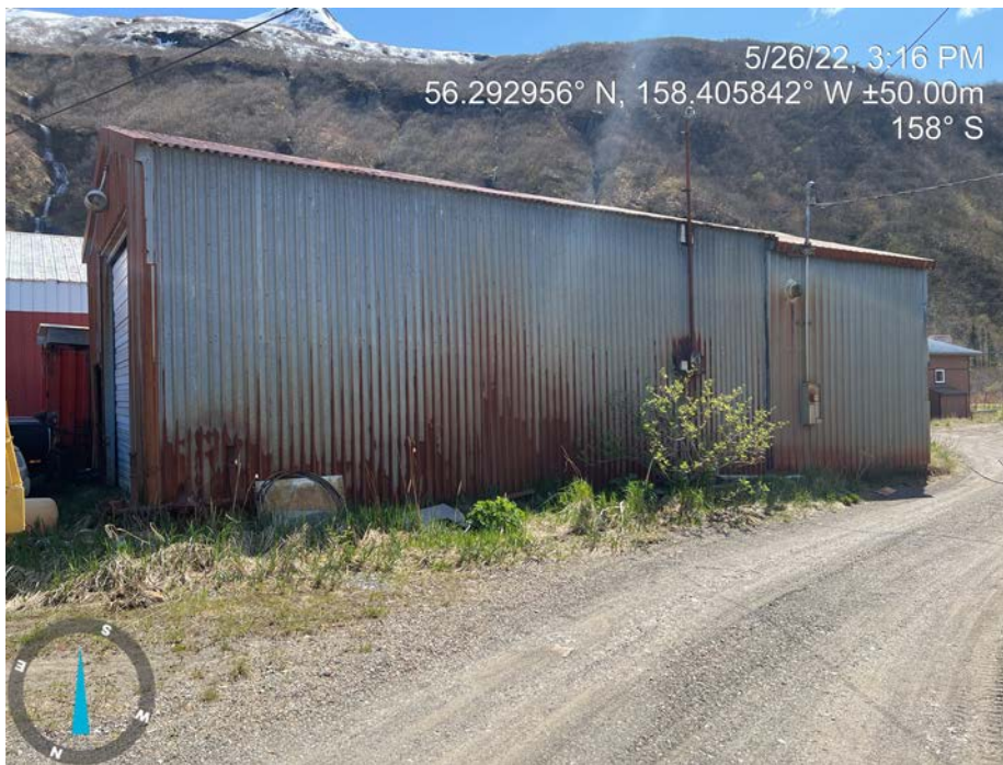
North Elevation 2 of 2
