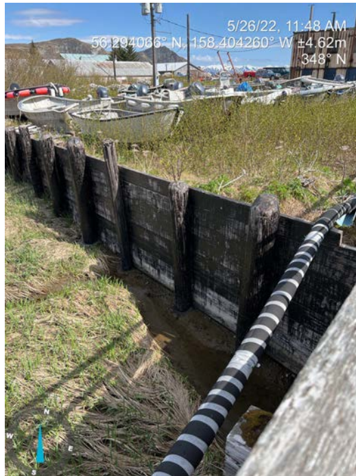
Retaining Wall on North Side
