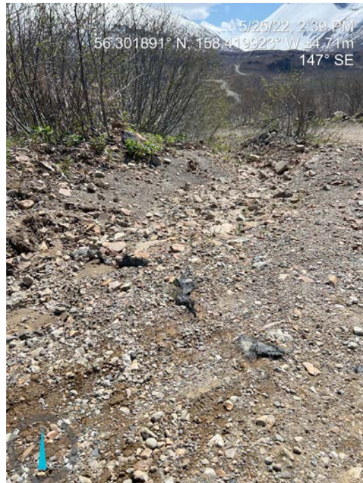
Exposed Geotextile
