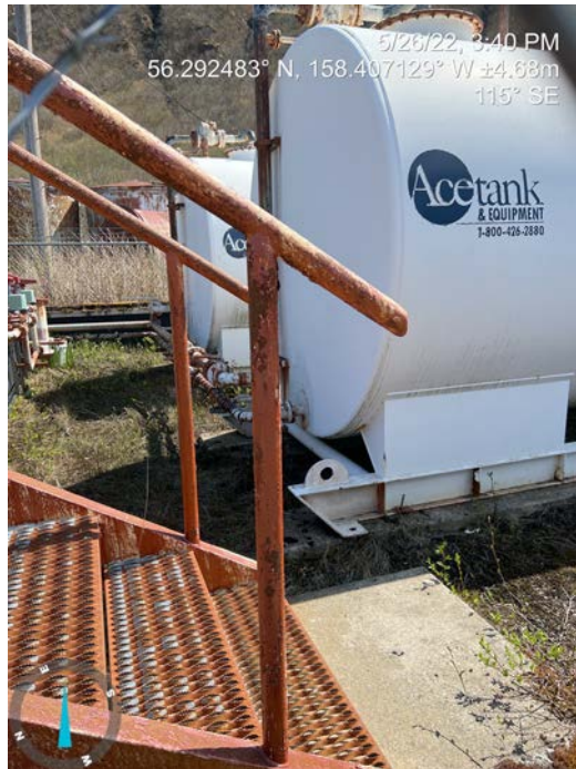
Metal Skid on Concret Planks
