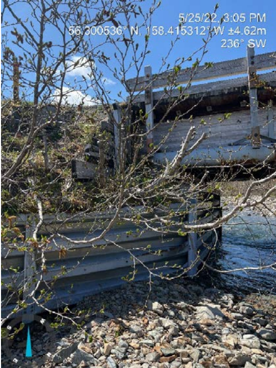
South Side Abutment
