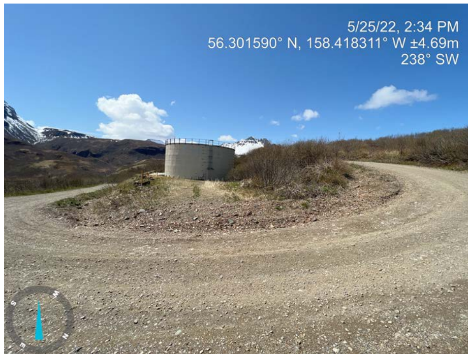
Lack of Ditching Around Bends 1 of 2
