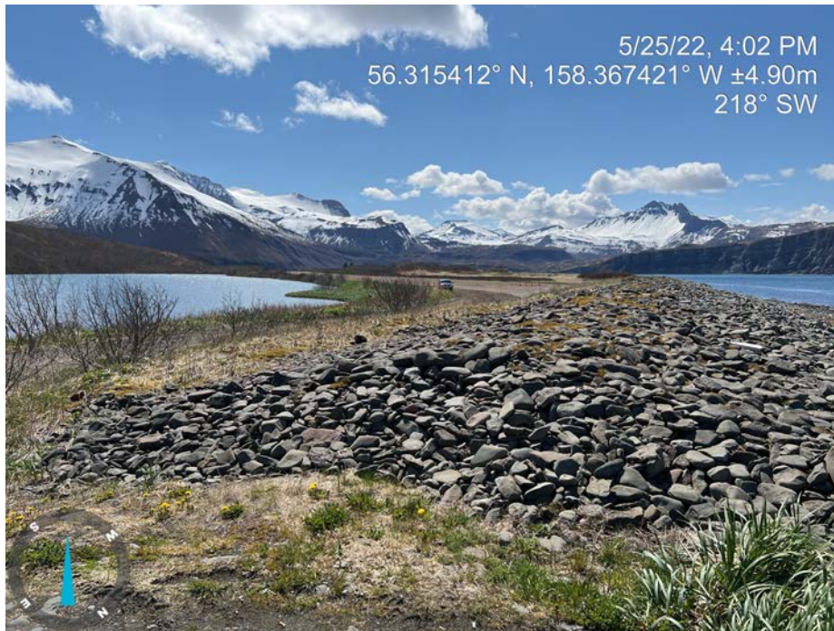
Runway Northeast Side 1 of 2
