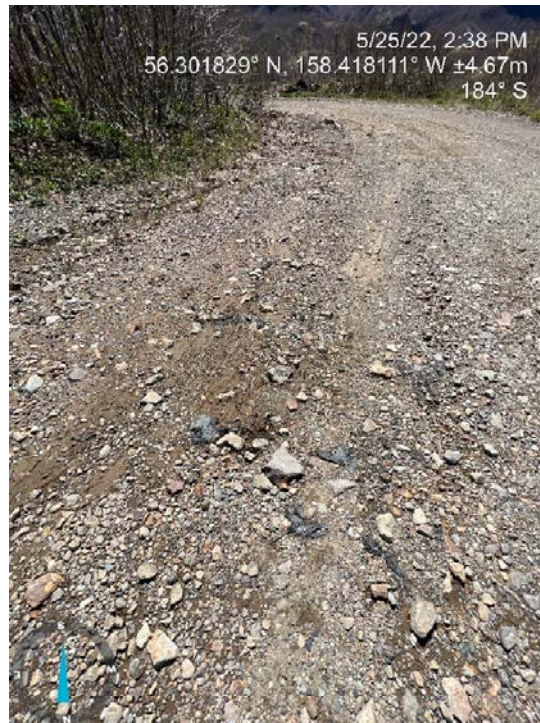
Exposed Geotextile
