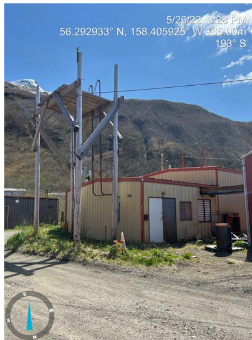
Wood Structure 2 of 2
