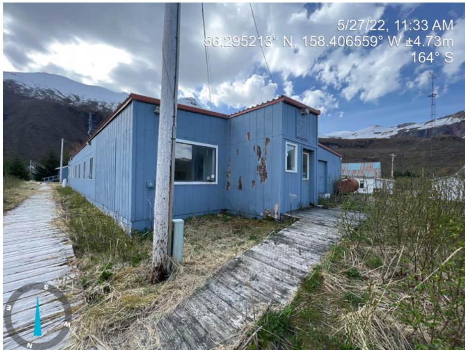
North Elevation 1 of 2
