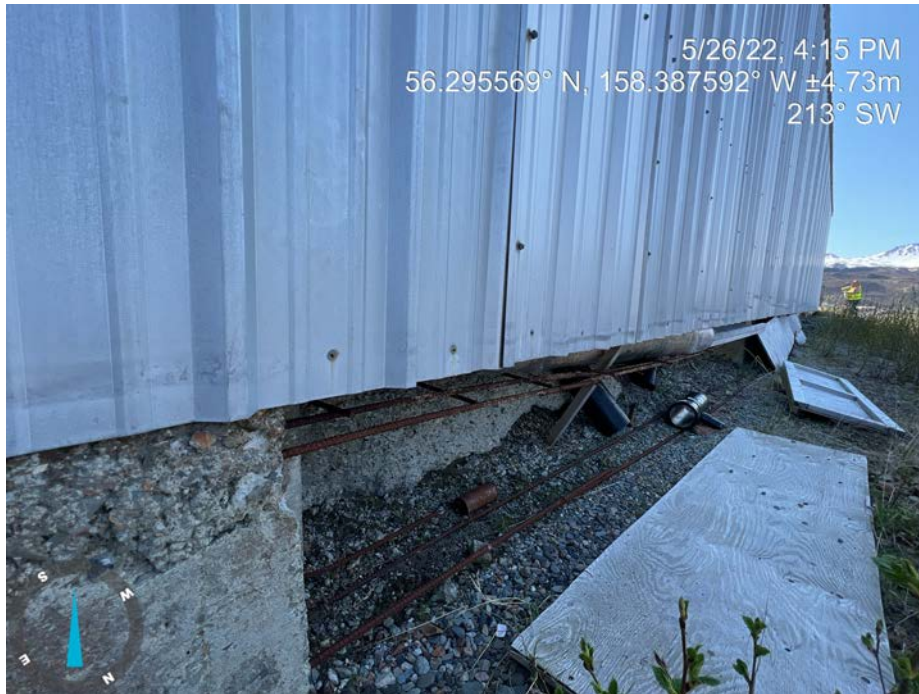
Damaged Concrete Foundation
