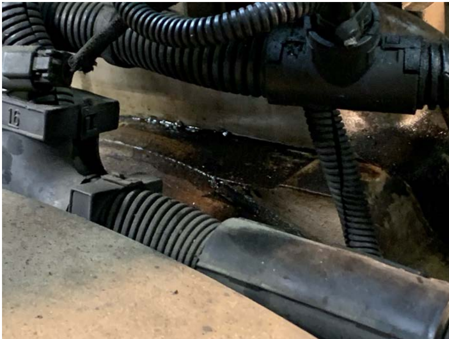
30 - #3 Engine Oil Leak
