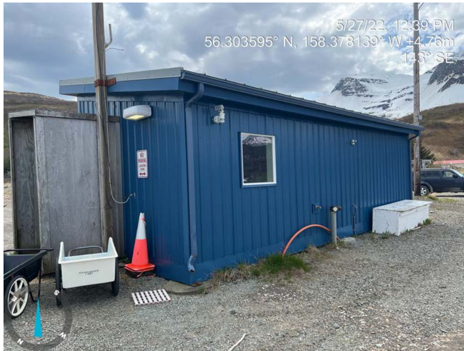
North Elevation 2 of 2
