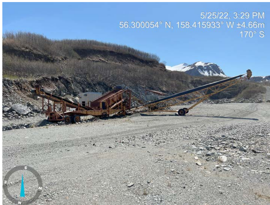
Rock Crusher 1 of 2
