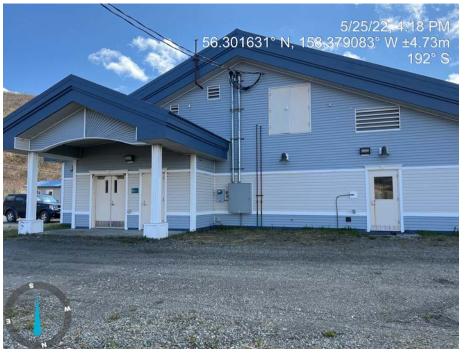
North Elevation 1 of 2
