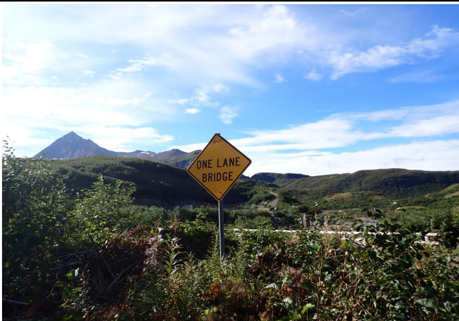
Bridge No. 1764 Br. Name Indian Creek Date 09/21/22 Inspector David McAdoo / Javier De Leon Frame 31 FE DS Sign File P9210420.jpg
