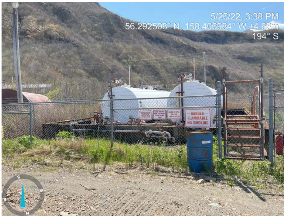
School Tank Farm 2 of 2
