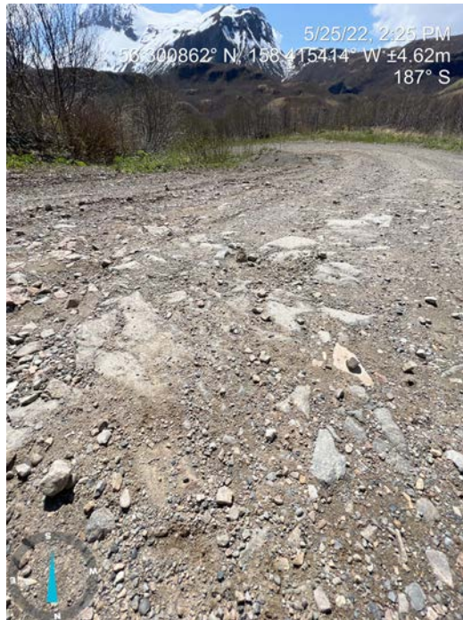
Runoff Washing Away Fines Exposing Larger Rock
