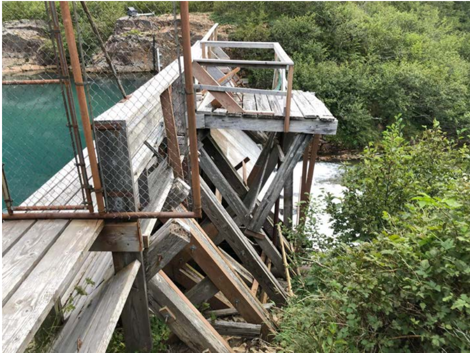
Indian Lake Dam
