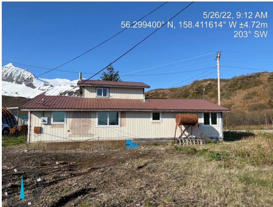
North Elevation 1 of 2
