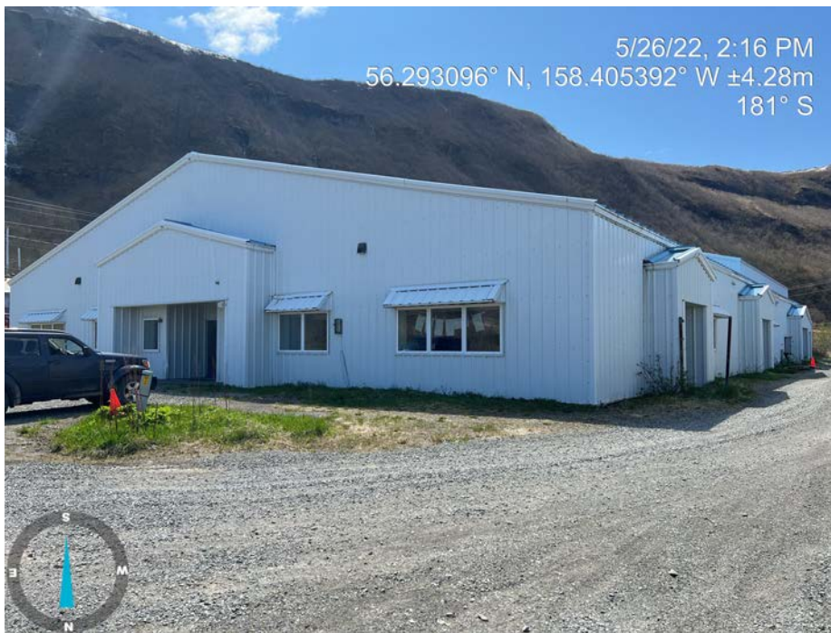
North Elevation 2 of 2
