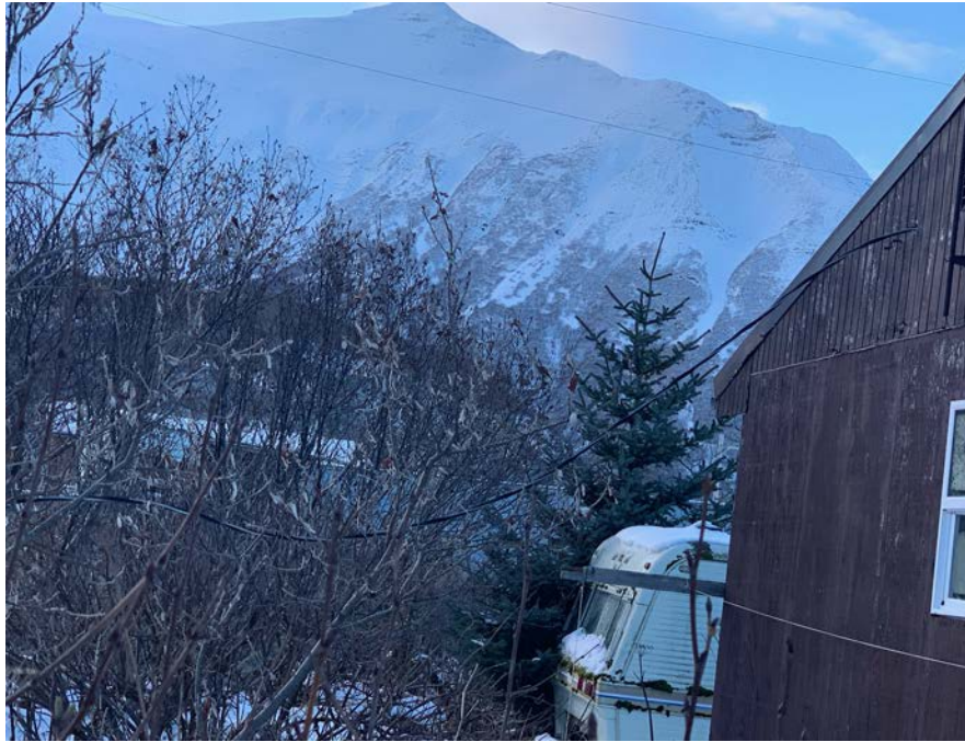
7 - Electric Service Line in Tree
